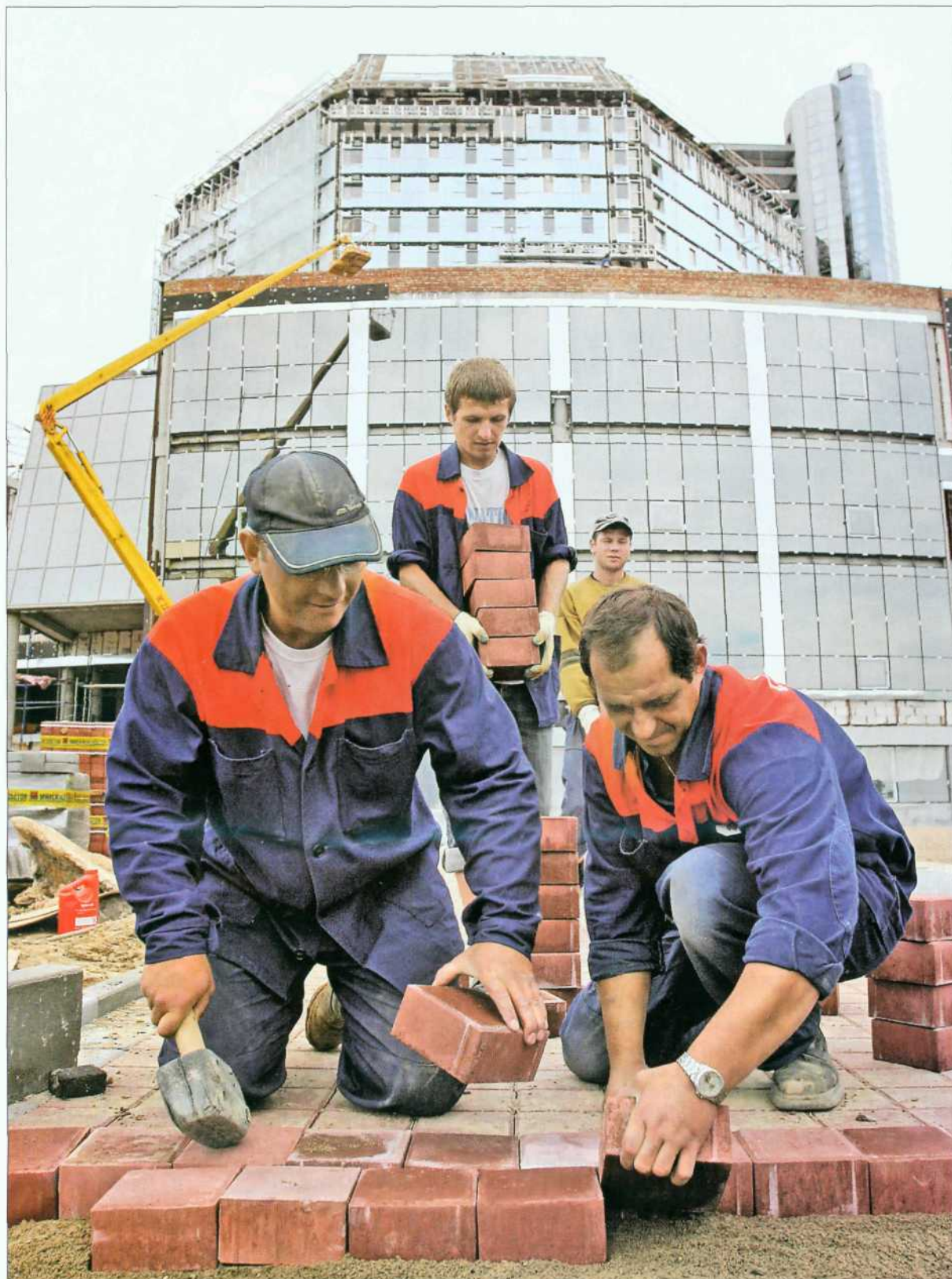
Construction of the new National Library approaches final stage
