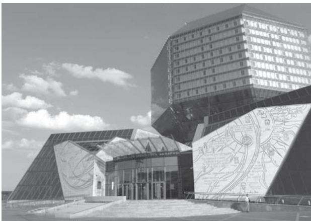
Figure 4. The main entrance.
