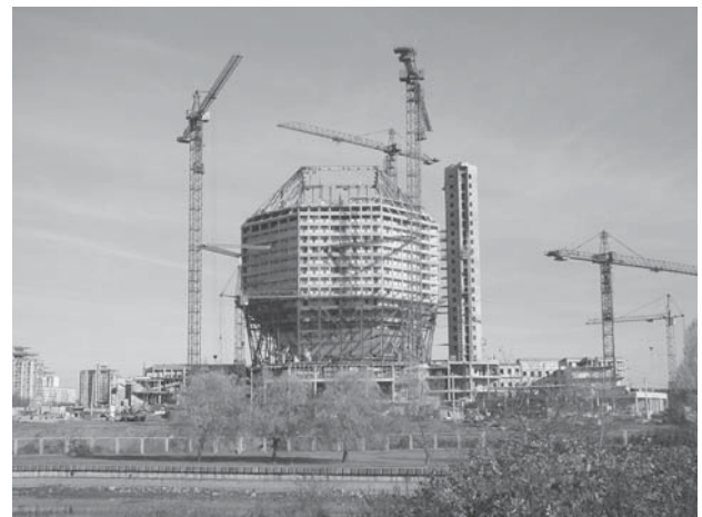
Figure 1. The Library under construction.
