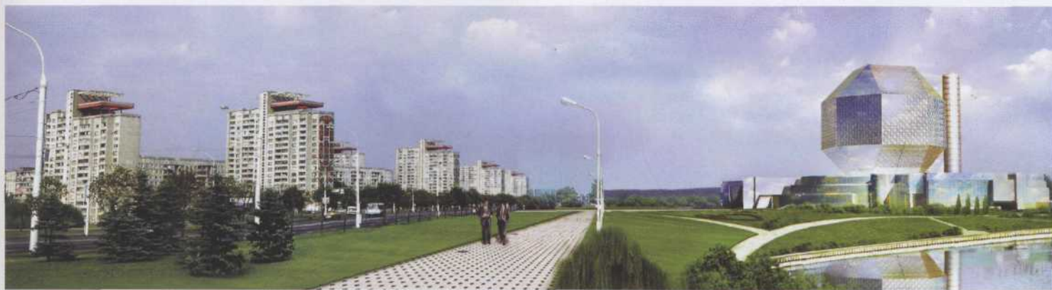
National library poised on its windswept site at the end of the Metro line.
